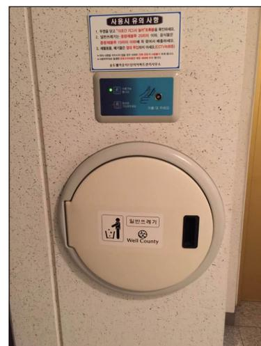
Fig. 5: The door in the staircase opening onto a pipe, which transports the domestic garbage on to the waste disposal plant.
